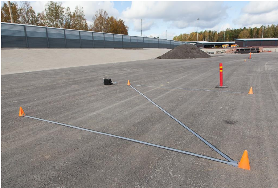
Figure 7. Coaxial cable-based traffic measurement installation on O-track. Photo: Mats Gustafsson, VTI.
